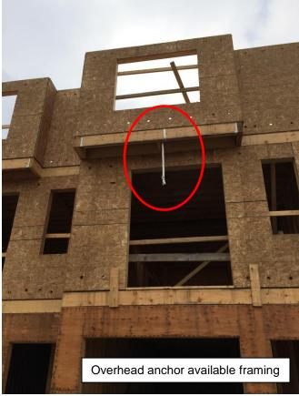
As shown in the photos, this anchor point will be available from the early stages of framing right up to the point where the final railing is installed. The anchor sling is wrapped around the header so it can be reasonably expected to serve as a Fall Restraint anchor point for the full construction cycle once installed.
