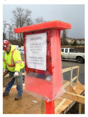
This fire extinguisher box is built to shed the rain and has a piece of poly protecting the opening. The poly can be easily removed to access the fire extinguisher (and air horn) for inspection and use.
