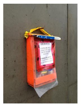
In a concrete tower or wood frame apartment it can be a challenge to maintain the location of fire extinguishers and air horns once the drywall starts going in the hallways. However, as shown in the photos below, sometimes the cut out for the final cabinet is the perfect size for the construction fire extinguisher and air horn.
