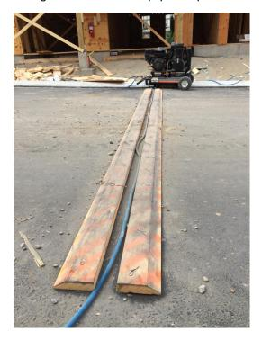
A 2x4 cord and hose path, pinned to the tarmac, protects equipment.
