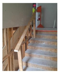
This photo shows a stairway handrail installed on the stairway risers several inches away from the framed wall. This allows the stairway wall to be substantially finished without removing the handrail. If the handrail does need to be removed temporarily then all that is required is to unscrew the posts from the stairway risers. The handrail can be quickly installed once the work is complete.
