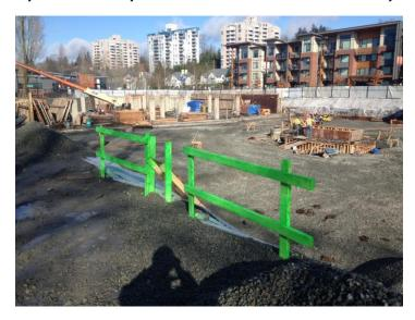
Adding the highly visible paint to this ladder access into an excavation makes it very obvious where the access point is.
